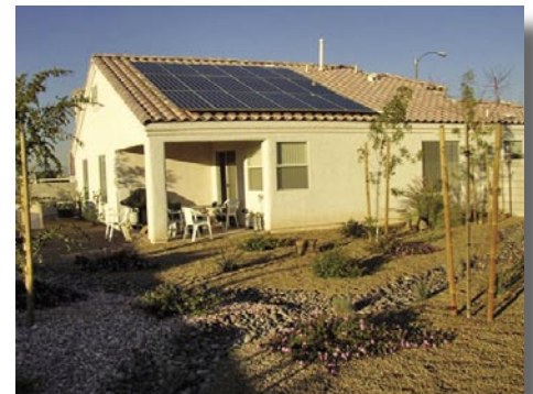
A SunWize Residential Grid-Tie System
